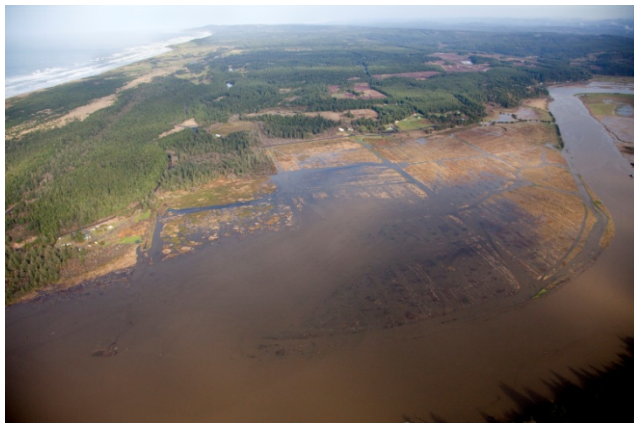
High tide aerial view of the Ni-les'tun tidal marsh restoration project, Nov. 2011, two months after the project was completed (Roy Lowe, FWS).
