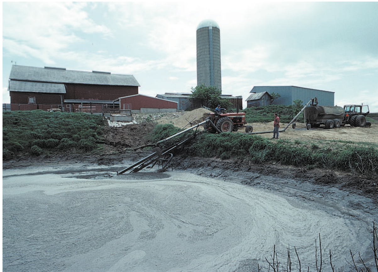
Liquid manure storage pit from a dairy operation in northeast Iowa., https://commons.wikimedia.org/wiki/File:NRCSIA99213 - Iowa (3121)(NRCS Photo Gallery).jpg
