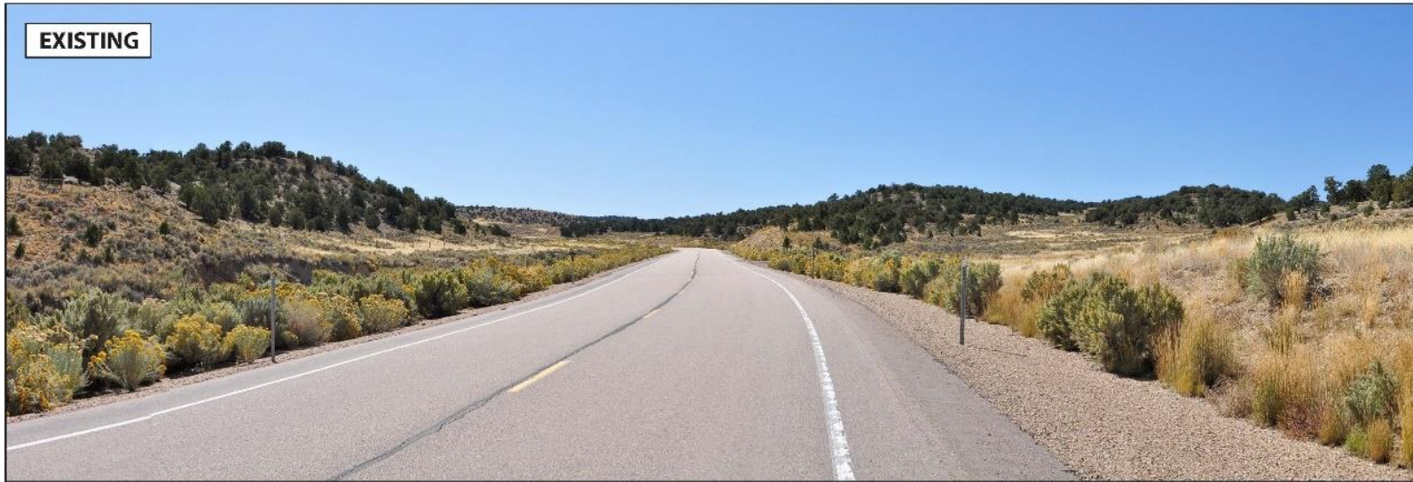
Figure 3.12-13-11. RKOP 037 Looking Southwest toward Grade-Separated Crossings at Milepost 61.06 and Milepost 61.00 (Wells Draw Alternative)
