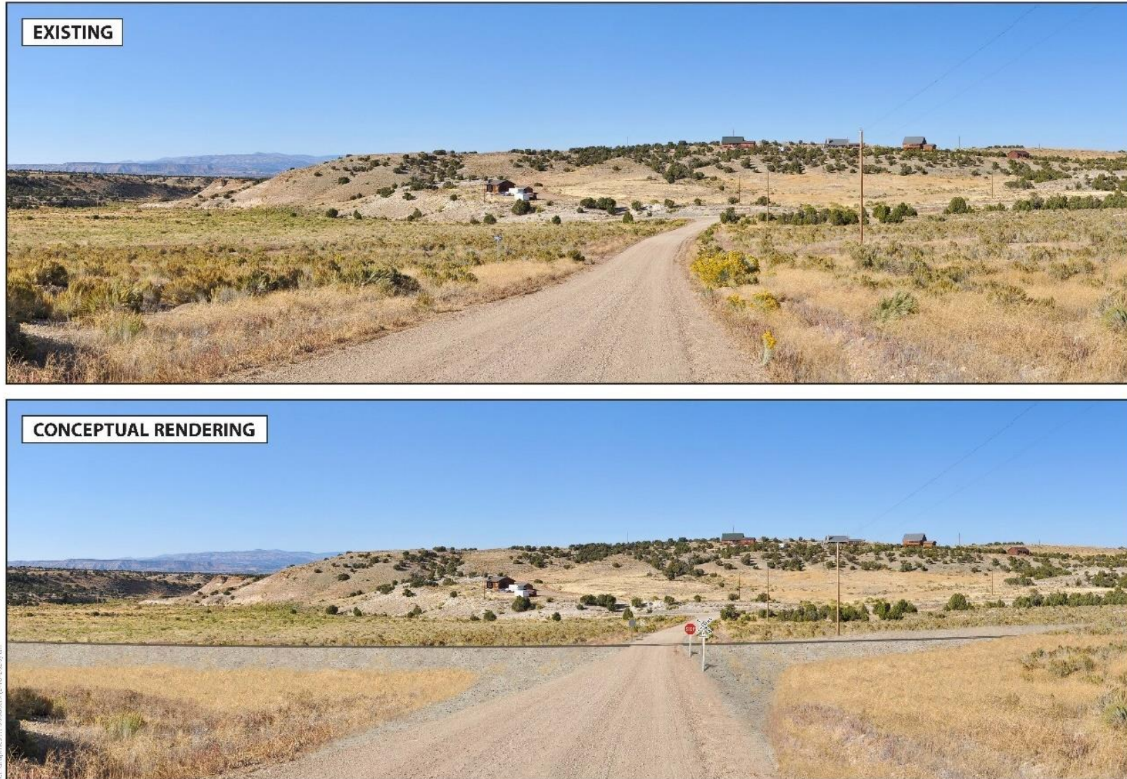
Figure 3.12-7. RKOP 146 Looking North near RC-Road Crossing at Milepost 50.50 (Indian Canyon Alternative)
