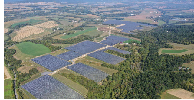
25 MW grid-scale system
