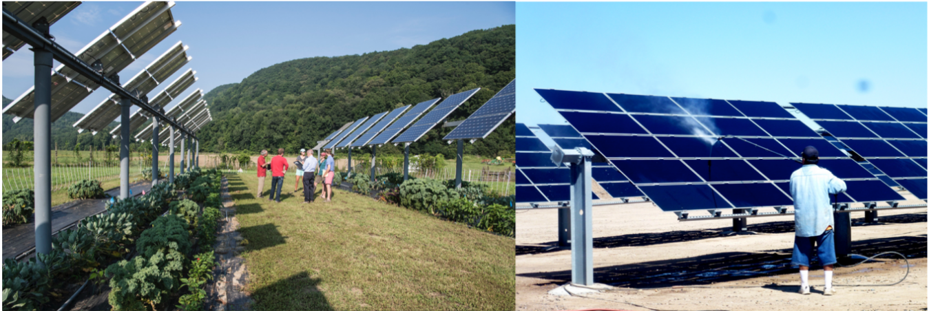
Figure 1 | Panel washing water inputs ( left ) are also inputs into agricultural productivity below (Center for Agriculture, Food and the Environment, University of Massachusetts-Amherst, South Deerfield, MA, USA photo: NREL) and panel washing ( right ) where water inputs are directed towards graded, compacted soil in California's Great Central Valley (Manteca, CA, photo: RR Hernandez).
