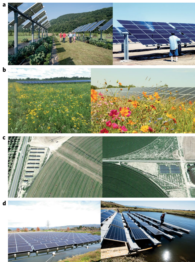
Fig. 3 | Techno-ecological synergies of solar energy and examples of techno-ecological synergistic outcomes. a , Panel washing water inputs (left) on a PV installation are also inputs into agricultural productivity below, known as an agrivoltaic system leading to increased water-use efficiency, erosion prevention and maintenance of soil fertility, land sparing and other beneficial techno-ecological outcomes (Center for Agriculture, Food and the Environment, University of Massachusetts-Amherst, South Deerfield, MA, USA). Compare this to panel washing (right) on an installation where water inputs are directed towards graded, compacted and barren soil in California's Great Central Valley, which does not optimize techno-ecological synergistic outcomes, like PV module efficiency of food system resilience (Manteca, California; for further discussion on water-use efficiency in agrivoltaics, see Supplementary Box 1). b , In the US states of Minnesota (left) and Vermont (right), land adjacent to croplands is developed with PV solar energy (1.3 MW, fixed tilt and 1.1 MW, single-axis tracking, respectively) and outplanted with low-growing flowering plants for native and managed pollinators that help increase agricultural yields, reduce management (that is, mowing) costs, and confer the opportunity to produce honey and other honey-based commodities. c , Centre-pivot agrivoltaic systems occupy the corners of crop/pasture fields for solar energy generation but also produce the techno-ecological synergistic outcomes of air pollution reduction, land sparing, food system resilience and others in Dexter, New Mexico (for further discussion on centre-pivot agrivoltaics see Supplementary Box 2). d , Floatovoltaic installations can contribute to local- and regional-scale agricultural resource needs while simultaneously enhancing water quality and water-use efficiency, a beneficial ecological outcome, as demonstrated by this floatovoltaic system in Napa, California (left) and this floatovoltaic system under construction atop a water treatment facility in Walden, Colorado (right; for further discussion on floating PV systems see Supplementary Box 3). Credit: Dennis Schroeder, NREL ( a left, d right); © 2018 Google ( c ); Greg Allen, Far Niente Winery ( d left)
