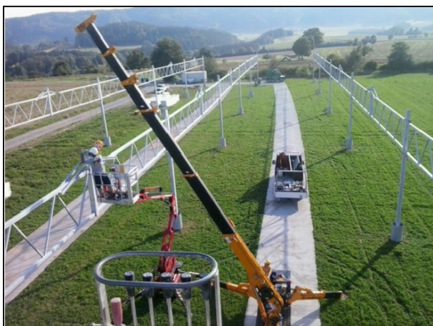
Fig. 4. (Left, source: BayWa r.e.): Installation of APV power plant with mobile soil protection panels in August 2016.
