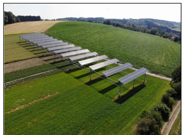
Fig. 6. (Left, source: BayWa r.e.): Scientific APV power plant from above with reference area next to it and in operation in 2018, producing Demeter-certified organic potatoes, winter wheat, clover, and celery.
