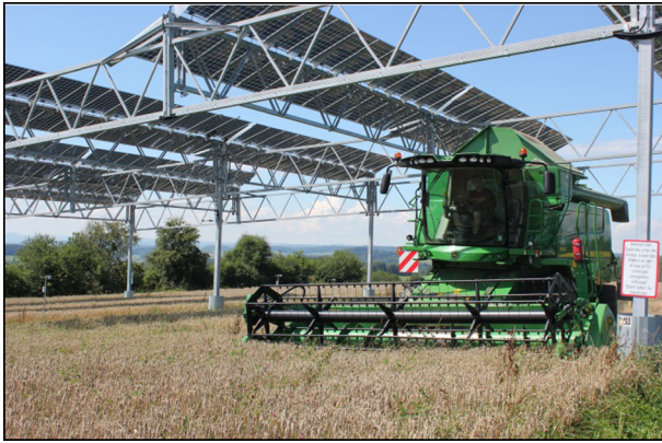
Fig. 7. (Right, source: farm community Heggelbach): Scientific APV power plant from above with reference area next to it and in operation in 2018, producing Demeter-certified organic potatoes, winter wheat, clover, and celery.
