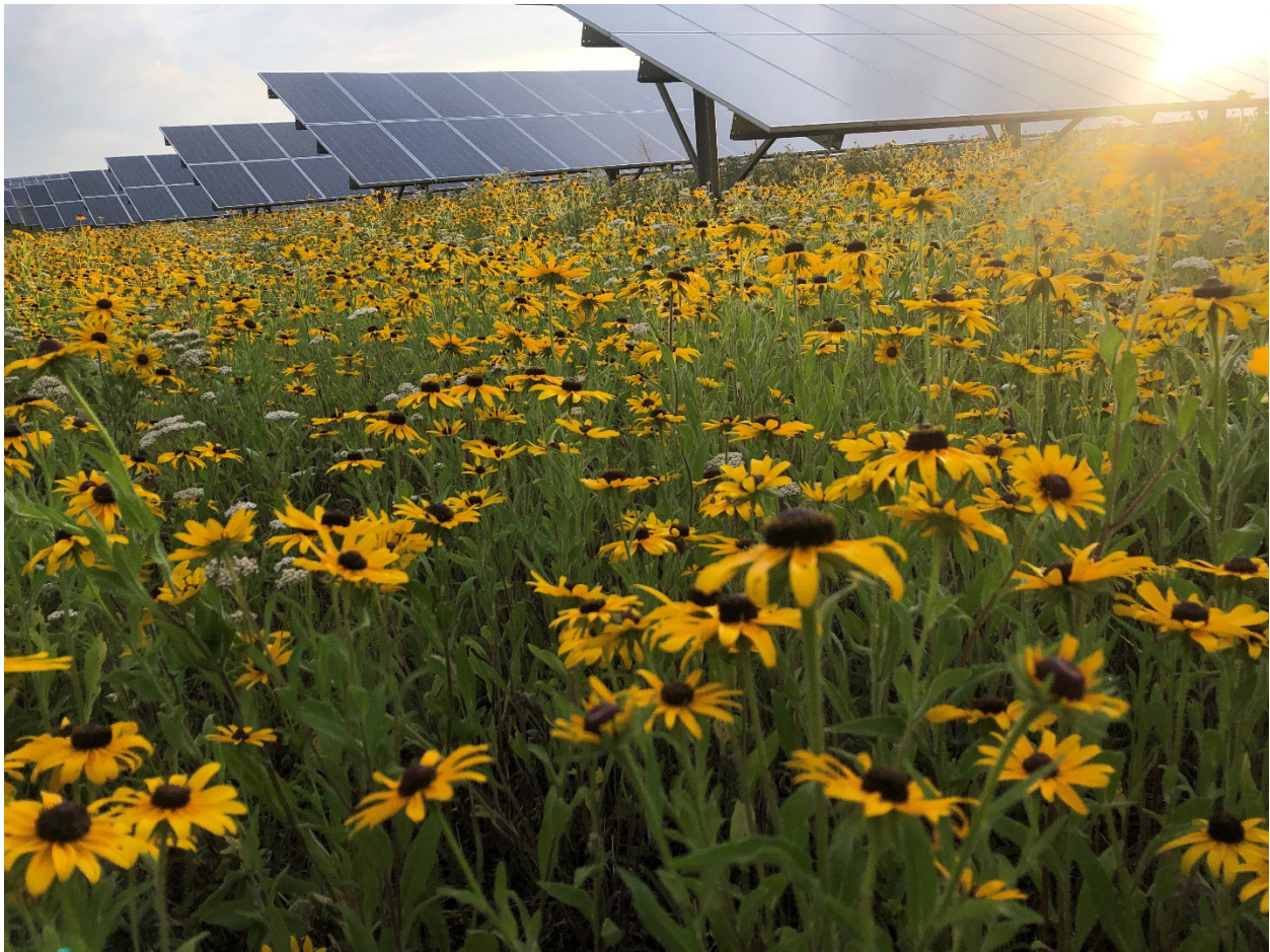
Figure ES-1. Connexus Energy solar array in Minnesota planted with pollinator-friendly groundcover
