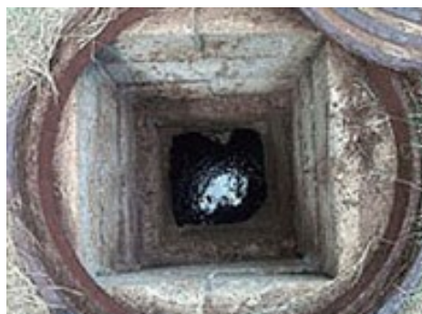
Figure 19: large capacity cesspool. Source GWPC
