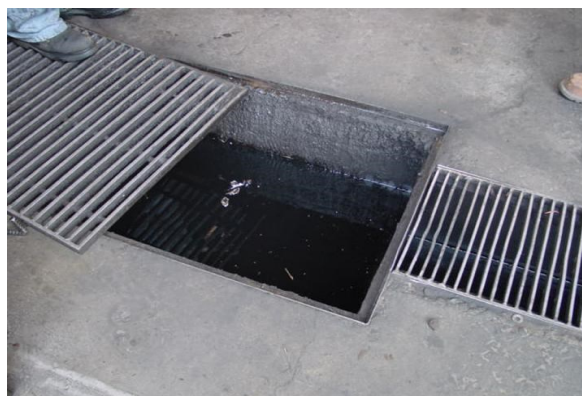
Figure 17: Typical Class V Motor Vehicle disposal well. Source GPWC
