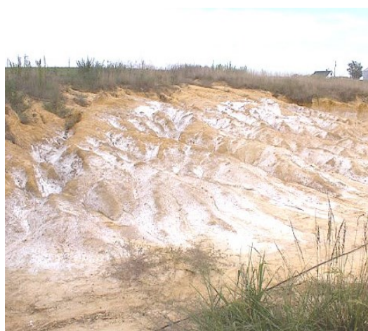
Figure 23: Produced water damaged soil: Source Southwest Indiana Brine Coalition
