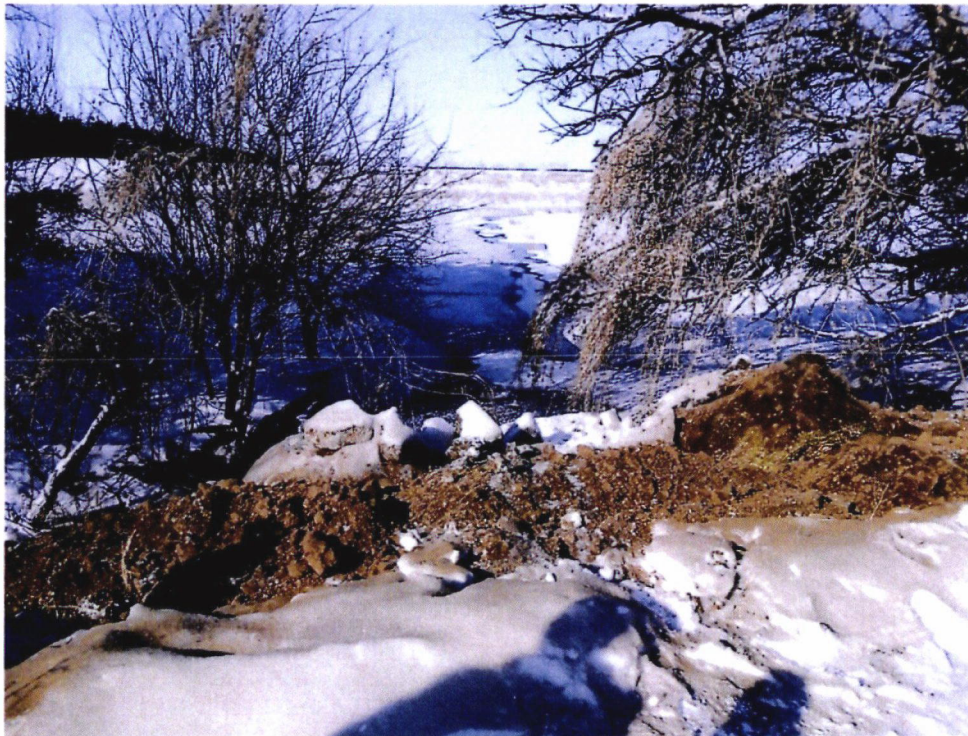
View WNW of dam upstream of culvert A
