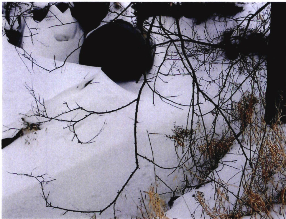
View east of upstream culvert inlet at Stop #2
