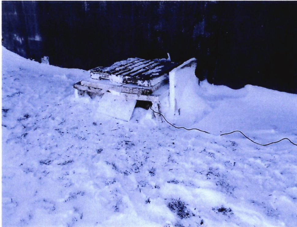
Insulation over piping vault on digester without leak
