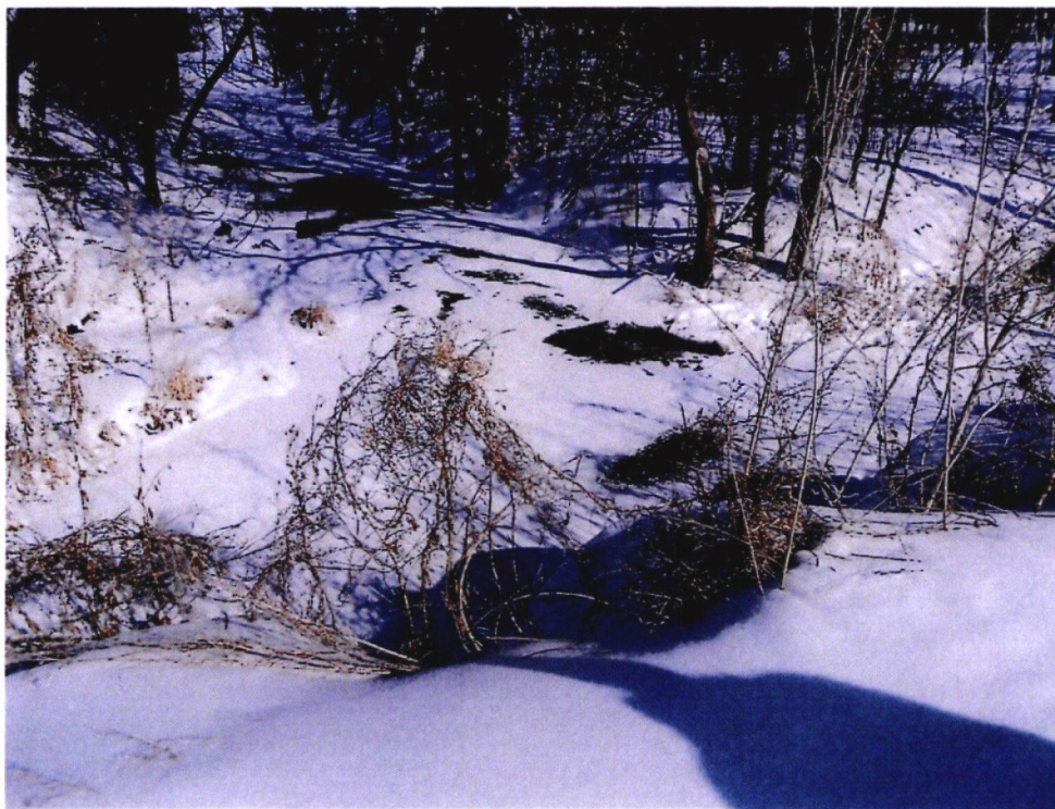
View north of ditch upstream from culvert D
