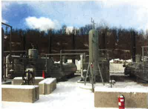
Figure 16. Gas-water separators at a HF well pad. Mouser photo.
