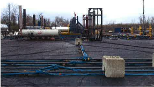
Figure 14. Surface piping moves flowback and produced fluids from the wellhead through gas-water separators to produced fluid tanks. Mouser photo.
