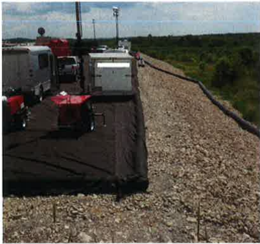
Figure 19. The edge of a well pad showing the pad height, edge slope, edge berm, and geosynthetic material. Mouser photo.
