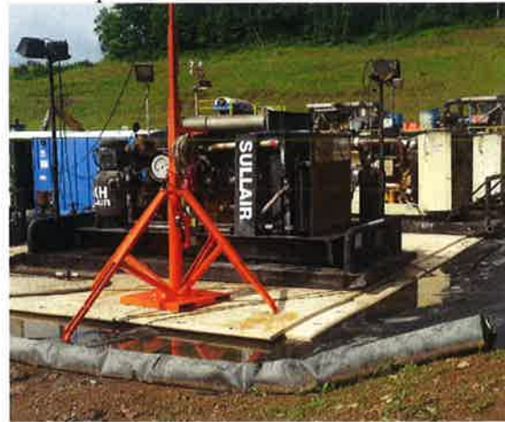
Figure 21. Equipment staged on a geosynthetic liner bermed at the downhill edges and covered by steel plates. Mouser photo.
