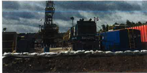
Figure 20. Equipment staged on a berm with a geosynthetic liner held in place with sand bags. Mouser photo.
