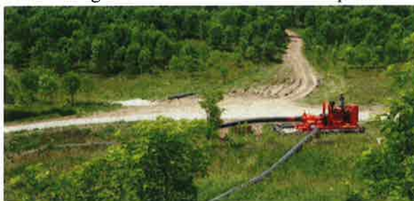
Figure 8. Water from the storage pond above is drawn using a gasoline-powered pump to storage containers on site. Mouser photo.
