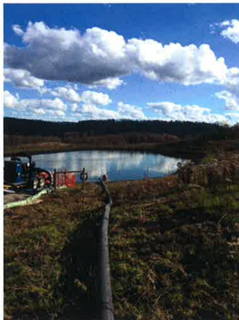
Figure 7. Water from a lined storage pond located off of the well pad is pumped through temporary piping for on-site drilling and HF activities. Mouser photo.
