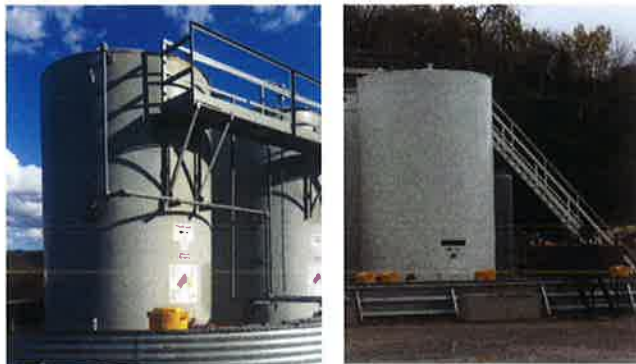
Figure 17. Permanent tanks storing produced fluids (left) or oil (right) during natural gas production. Mouser photo.
