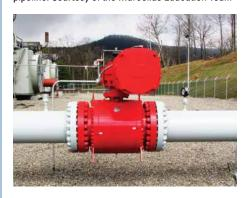
vent compressor station gas piping (sometimes referred to as a blow down). Regulations require that compressor stations periodically test and perform maintenance on the emergency shutdown system to ensure reliability. It is advisable for landowners, neighbors, and first responders to become familiar with safety systems, testing procedures, and emergency response protocols for compressor stations in their area.
