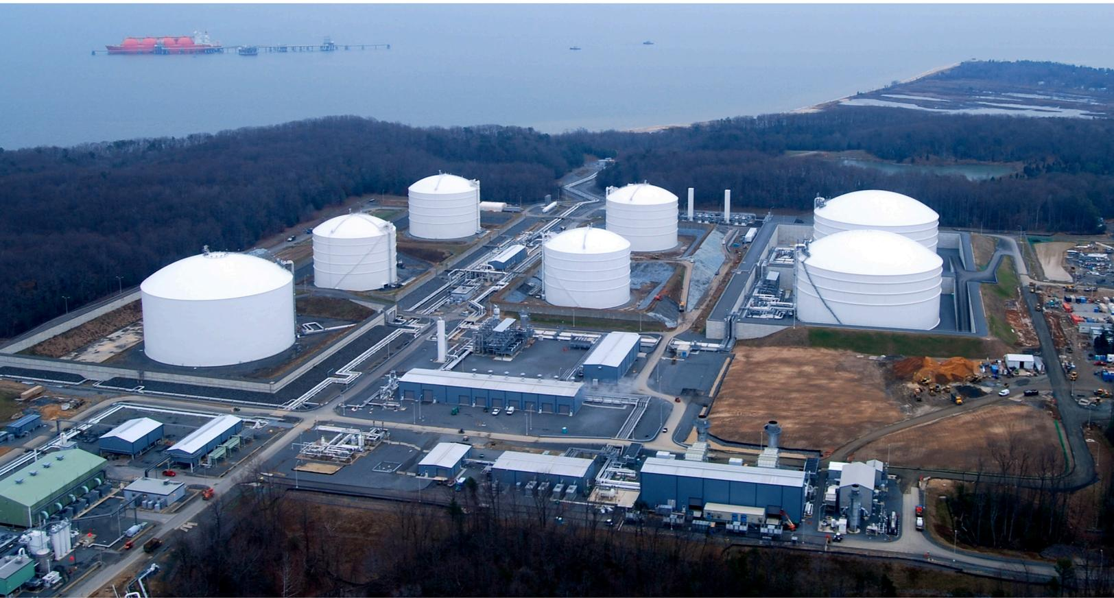
LNG, or liquefied natural gas, is a clear, odorless, noncorrosive, nontoxic liquid that is formed when natural gas is cooled to around -260 F. This shrinks the volume by about 600 times, making the resource easier to store and transport through marine shipments. LNG is not stored under pressure and is not explosive or flammable in its liquid state, and it cannot be released rapidly enough to cause overpressures associated with explosions.
