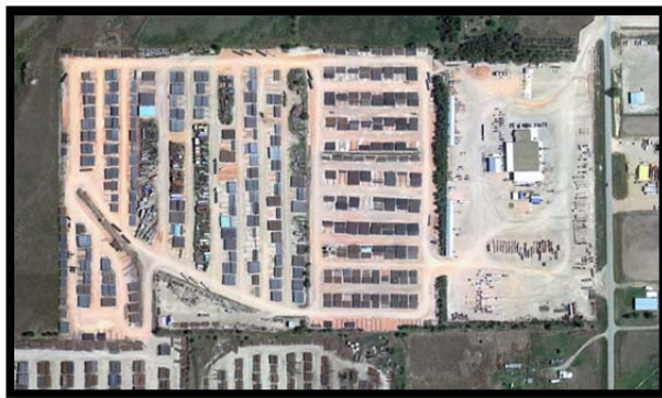
Figure 23: Typical Construction Staging and Equipment Areas (Photo courtesy of Robert M. Donnan, http://www.marcellus-shale.us/ )
