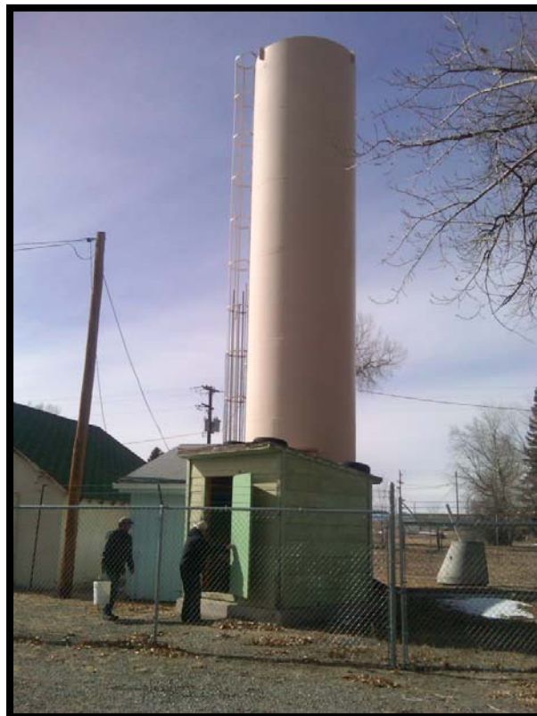
FIGURE IV-6: Stand Pipe Tank
