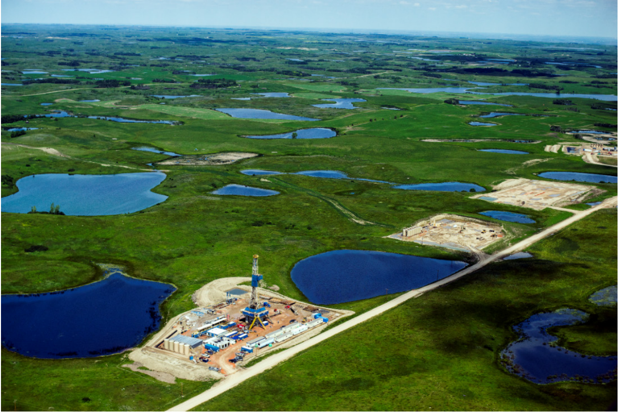
Figure 3-10. Aerial photograph of hydraulic fracturing well sites near Williston, North Dakota. Photo credit: Image@J Henry Fair / Flights provided by LightHawk.
