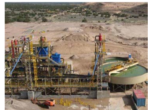
Victory Nickel – Frac Sand Processing Plant Minago, Manitoba, CA
